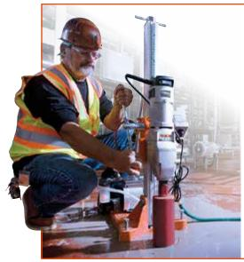
Core bits are cutting tools used to remove a cylindrically shaped piece of material. A core drill is designed to cut a hole and remove a core sample or to drill a hole without leaving material behind. Diamond core bits have diamond cutting tips and are frequently used for drilling in materials such as concrete, stone, and asphalt.
