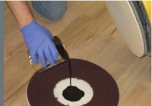
Step 1 - Cut in edges, load pad with stain
