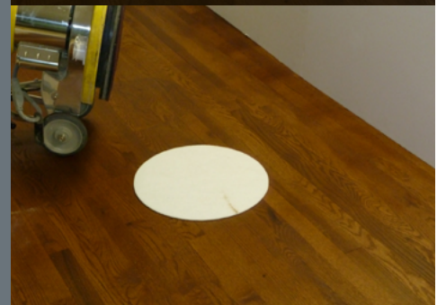
Step 3 - Replace stain filled pad with clean pad
