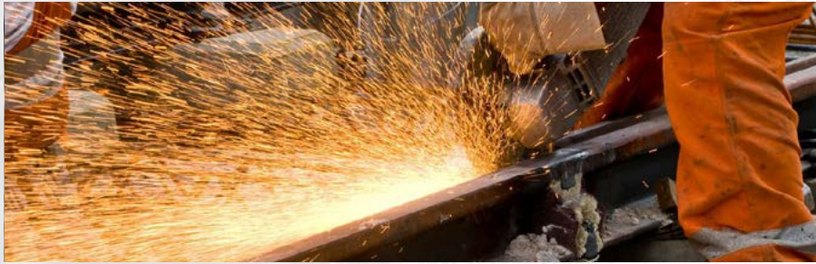
Straight and recessed organic wheels for grinding Frogs and Switch Points
